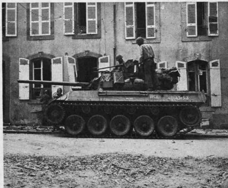
Star performer in France has been the M-18 with its 76-mm. weapon and top speed of 55 m.p.h. It was the first U. S. armored vehicle with the modified Christie running gear ( see M-19 opposite ) to go into action.
